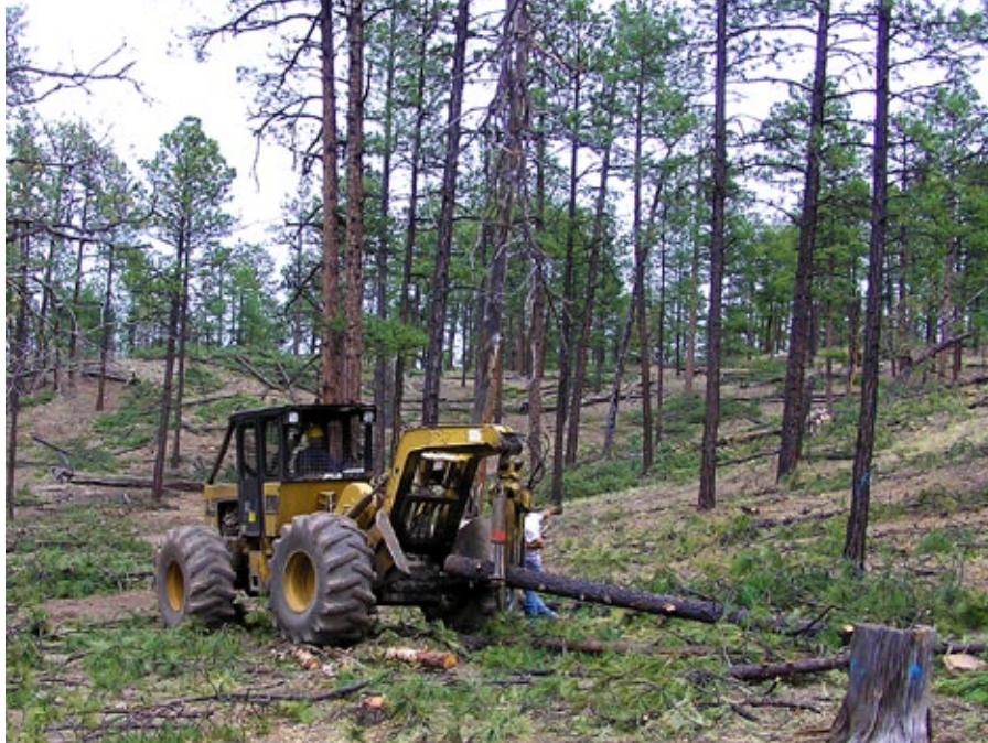
Using a skidder to remove small-diameter trees.
